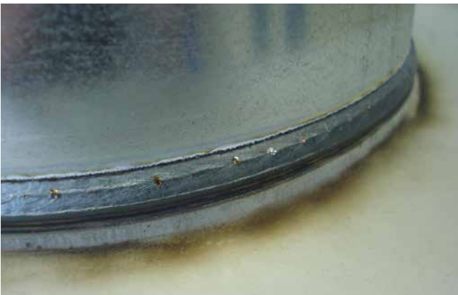
Welding galvanised sheet metal
