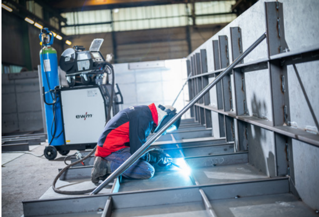
Every day, Heinrich Döpke GmbH welds up to 22 meter long components made of black and stainless steel. For this purpose, they have been using the modern EWM Titan XQ 350 puls welding machines with wire feeder and EWM PM 451 welding torch since 2020.
