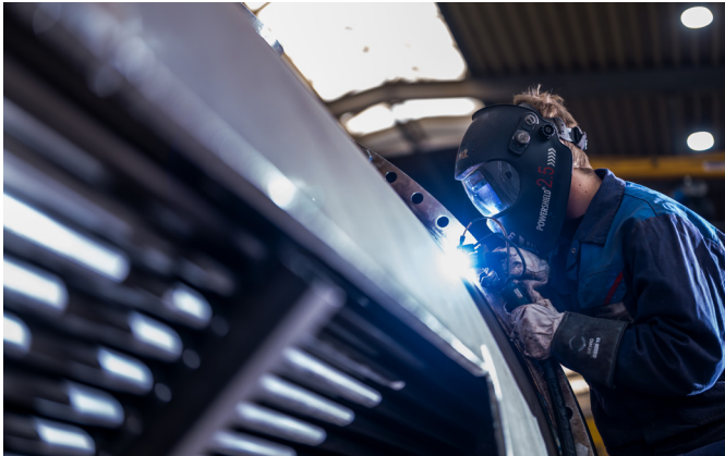
Welding a heat exchanger flange made of P265 GH with a diameter of 2.30 meters using the tigSpeed system.
