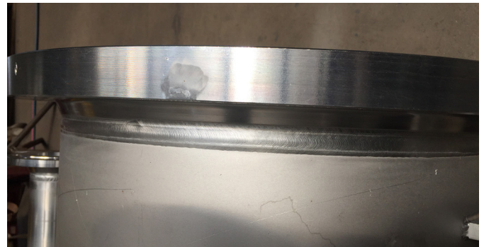
Completed weld on a flange pipe connection of a duplex steel container
